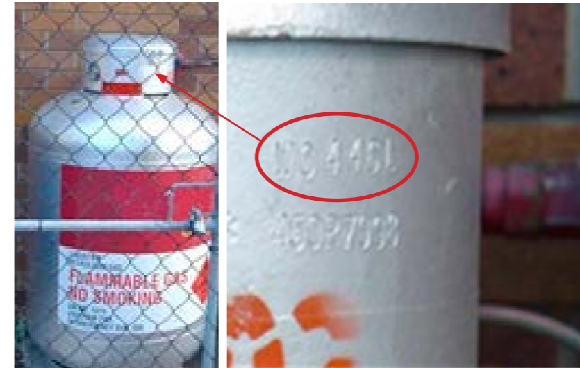
Figure 5. Gas cylinder and a close-up view showing 'water capacity' (WC) value
